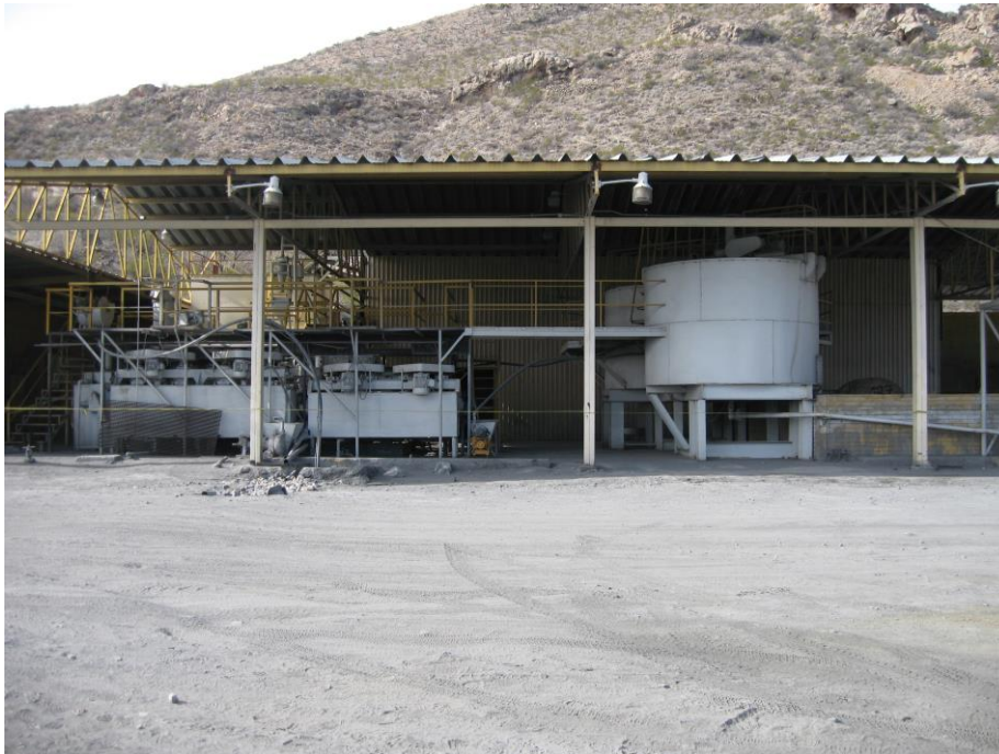
Figure 1: The Plomosas processing plant before refurbishment
