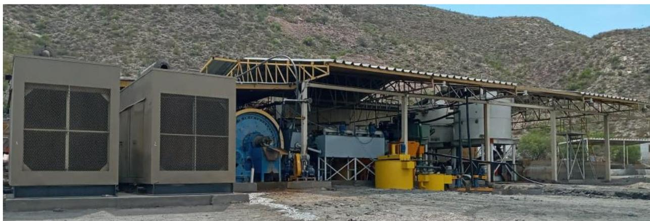
*Picture 1: Completed processing plant – reconditioned mill, power supply, float cells and thickeners.*
